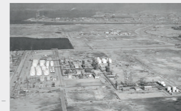
Nissan Petrochemicals Chiba Plant (1968)
